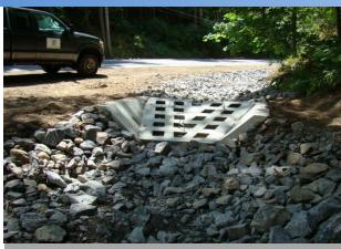
Sediment basins help to reduce the amount of sediments that enter our water sources. This one was installed in the summer of 2016 (top), and was tested out in some spring thawing February 2017 (bottom)!
