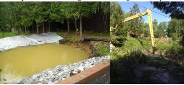
Pictures to the left show the pond being worked on to help keep water clean. The rerouted drainage system to the right is now stable and keeping water clean.
